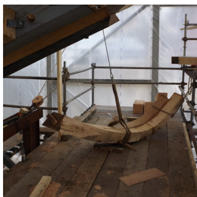
One of the starboard frames ready to position, notice the tenon that will be inserted into the mortise.
